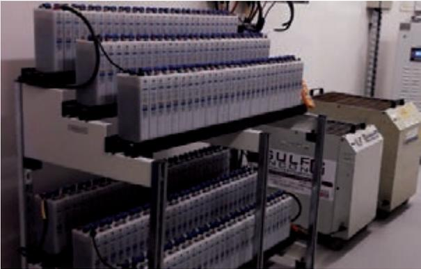
Discharge testing is the only test method that provides a comprehensive insight into battery capacity, and is therefore an essential part of vigorous battery maintenance programmes. Load testing is used to verify that the battery can deliver its specified power when needed.
